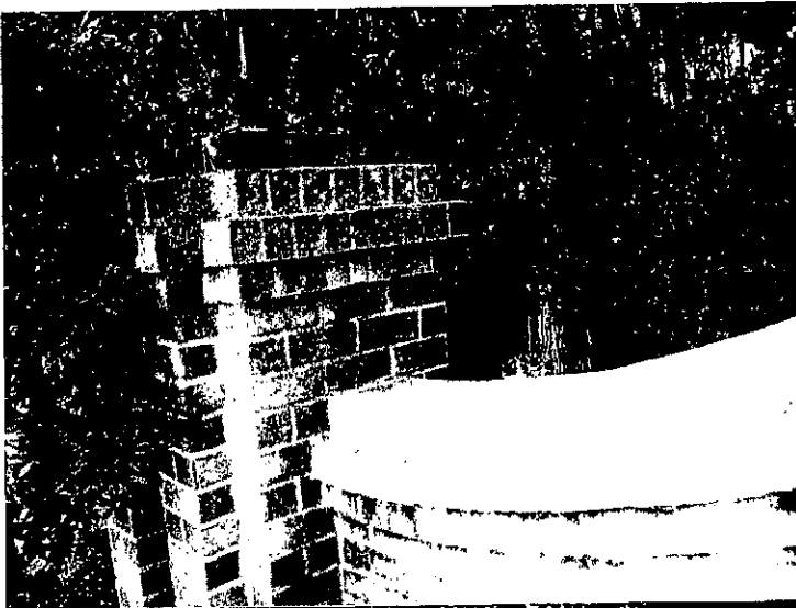
Photo #4: There is vegetation growing very near the monument brickwork. This can damage the brick by abrasion in wind and by retention of moisture. There is Leichen growing on the brick also. It is advised to clean the brick and trim back vegetation before these cause premature degradation to the wall.
