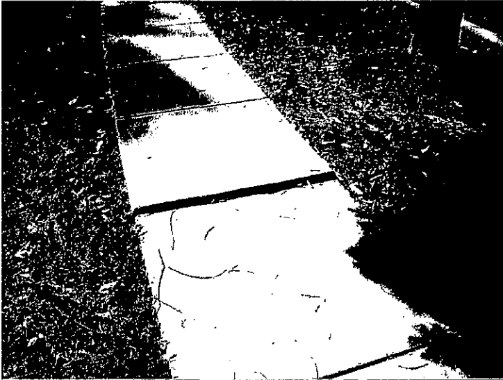
Photo #2: Across Hawkesbury Lane from 719, the sidewalk is out of alignment in several areas by some 2" causing a trip hazard. It is advised to shave down or replace the areas that are out of alignment. (Public Sidewalk)
